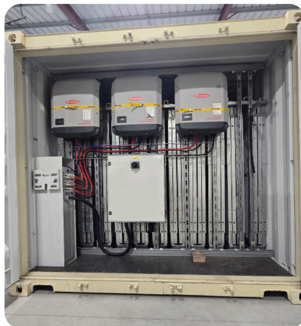
Container On-grid with conversion unit
